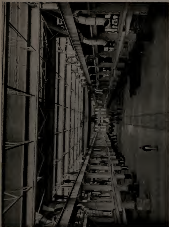
Typical Layout of Piping Showing Main Ducts and Branch Outlets, as used with Fan System Heating Apparatus in a Machine Shop
